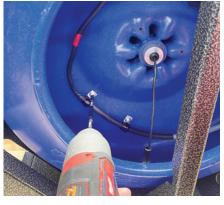
Remove the two brackets that secure the end of the old push-rod to the reel.
