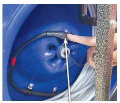
Carefully cut the membrane wrap on the push-rod side and peel back.
