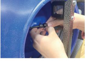
Without wasting time and working while the membrane is pliable, position the last 2 clamps over the membrane on either side of the connection.
